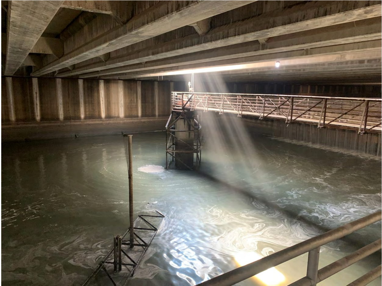
Figure J-4: Flow Equalization Basin in PTC 2
