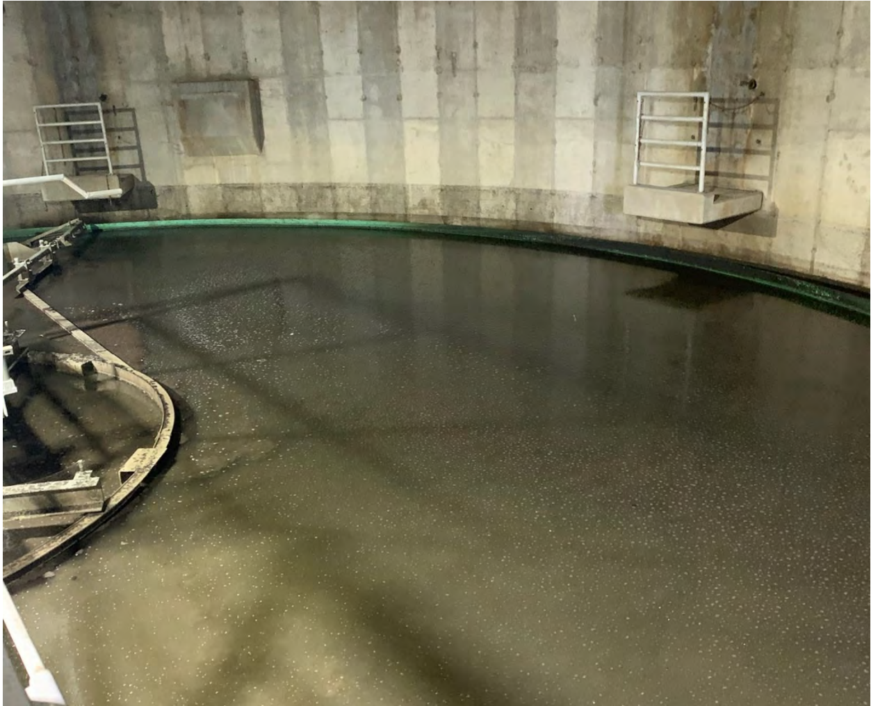
Figure J-11: Gravity Thickener
