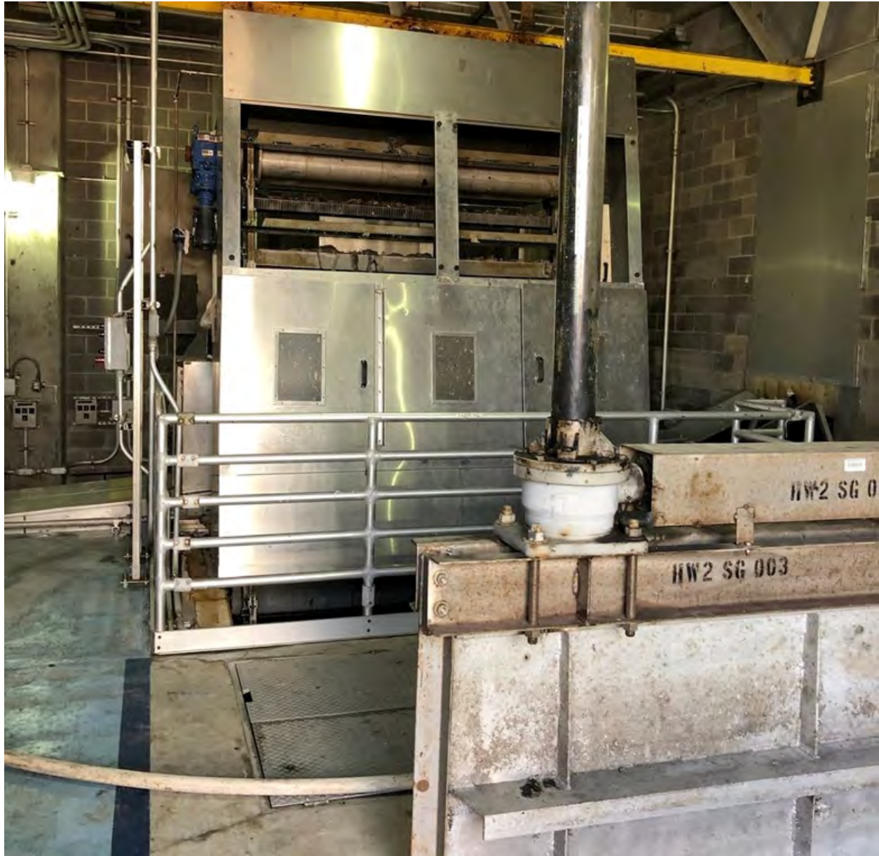
Figure J-1: Coarse Screen in HW 2
