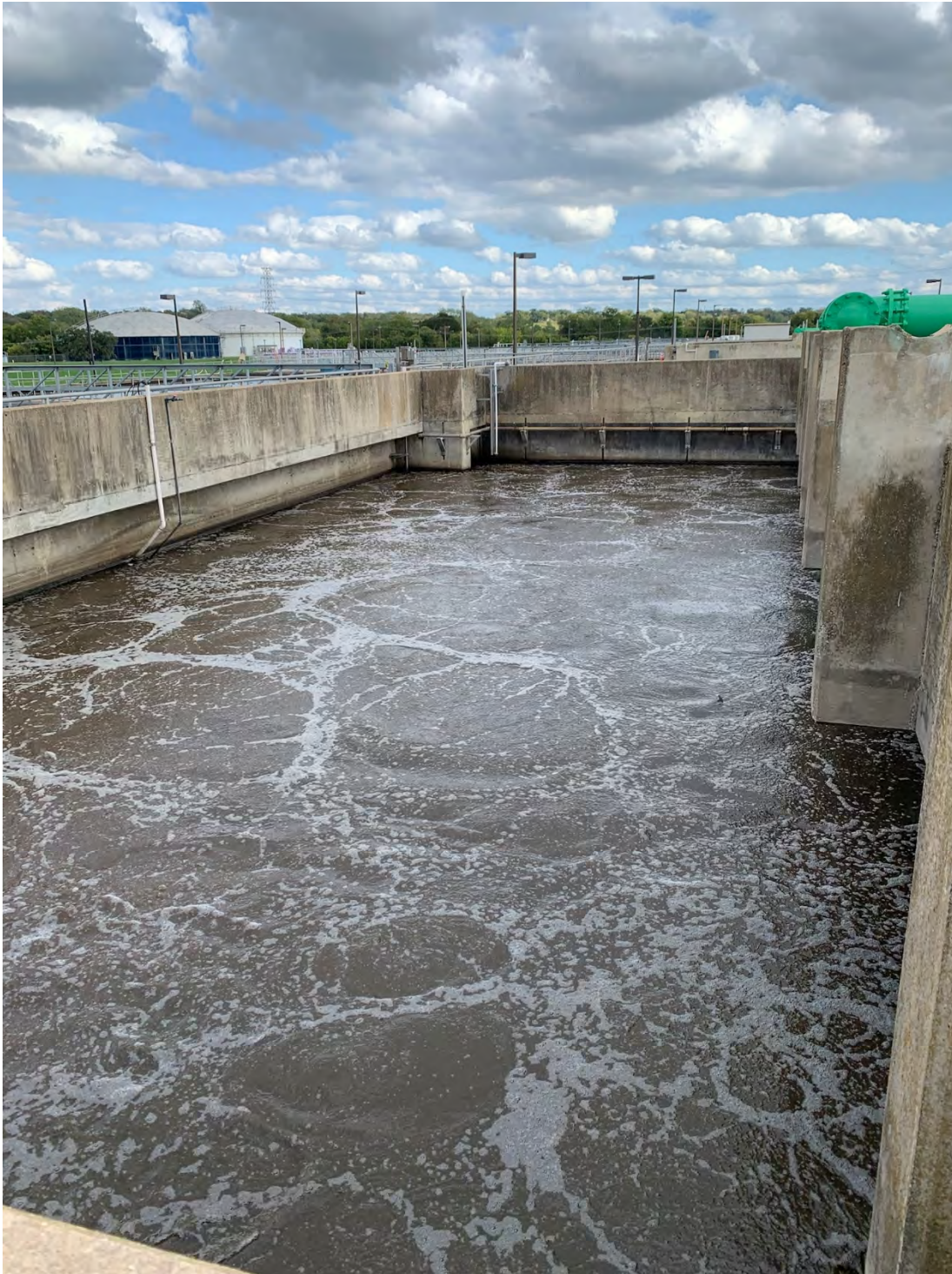
Figure J-7: Flocculation Basin in ASC 1
