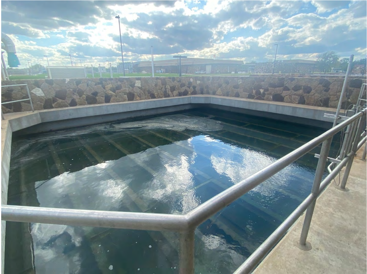
Figure J-10: Gravity Filtration Unit
